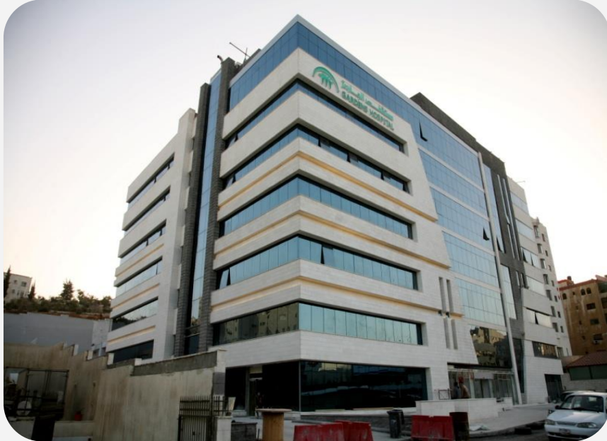
Al Gardenz Hospital
